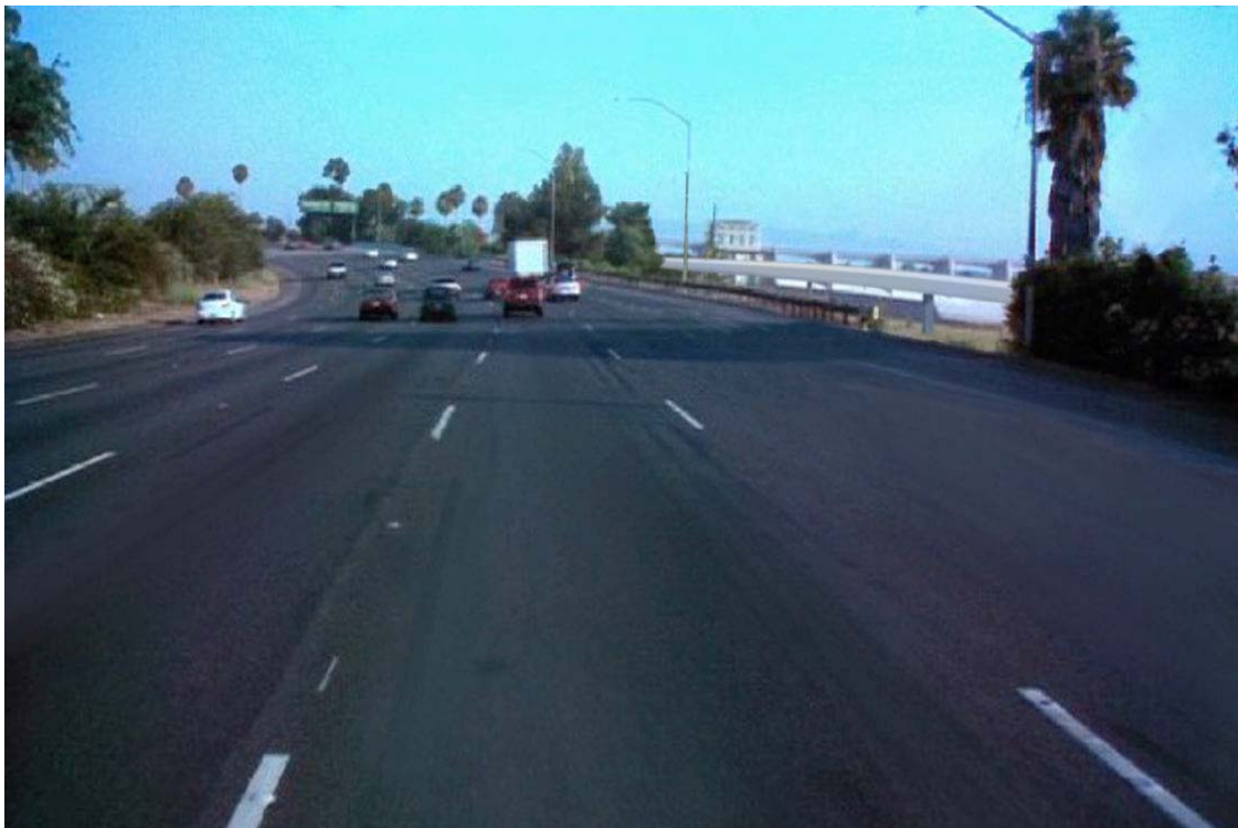
Figure 26b. Viewpoint 7 – Existing View Facing Northwest on US-101 at Sepulveda Dam with Post-Construction Simulation
