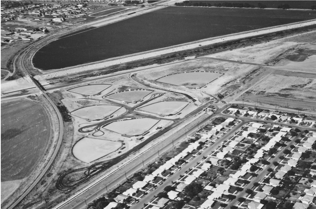
Sepulveda Ball Park Being Constructed, June 1955
