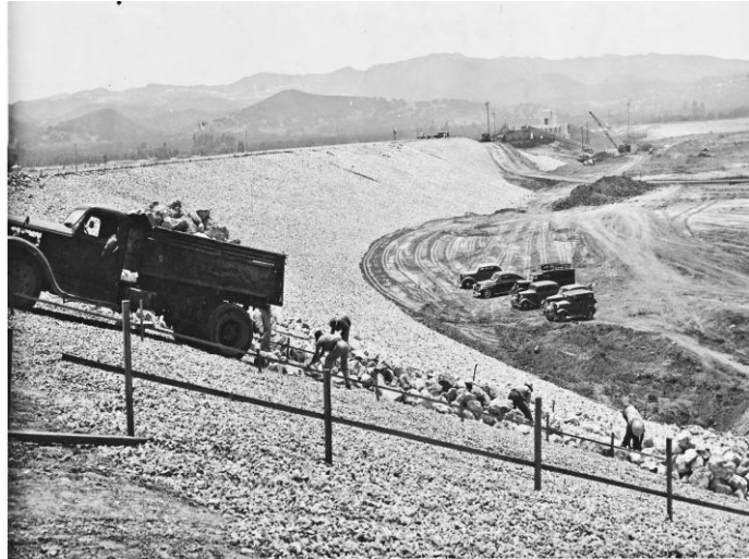
Sepulveda Dam Construction 1940
