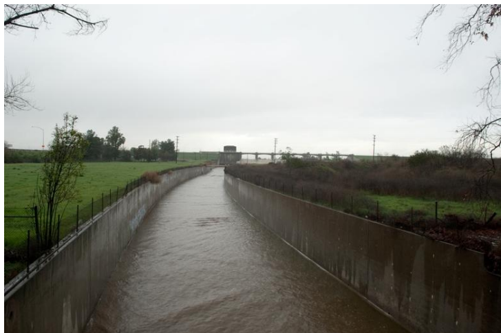
Sepulveda Dam and Channel
