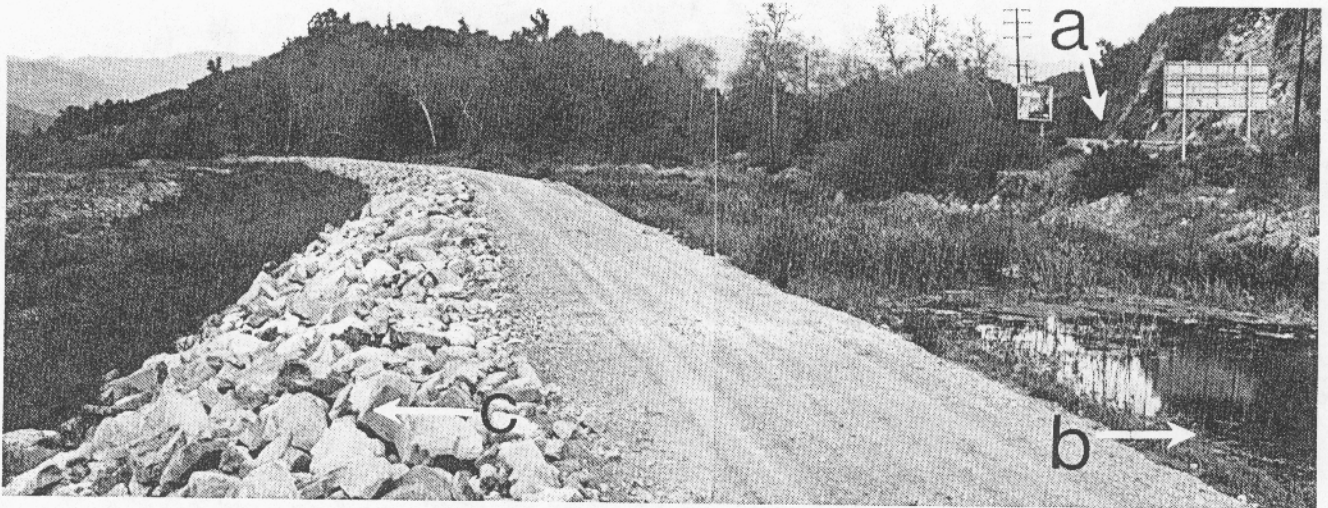
Figure 5.--Separation of riparian areas: a) Highway 33; b) isolated area with ponding water and cattails; c) levee built in 1978 in the Ventura River just downstream of its confluence with San Antonio Creek. (Photograph taken in March, 1981).
