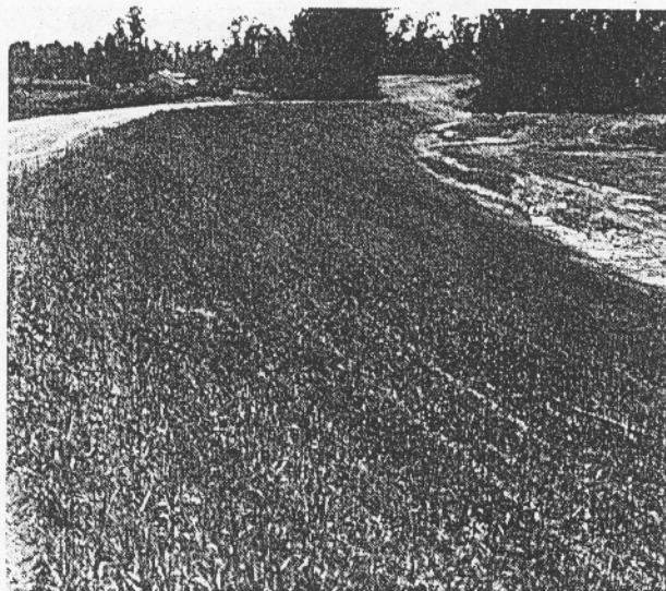
Figure 6.--Flood retention dam, Sycamore Canyon Dam, Simi Valley, California.
