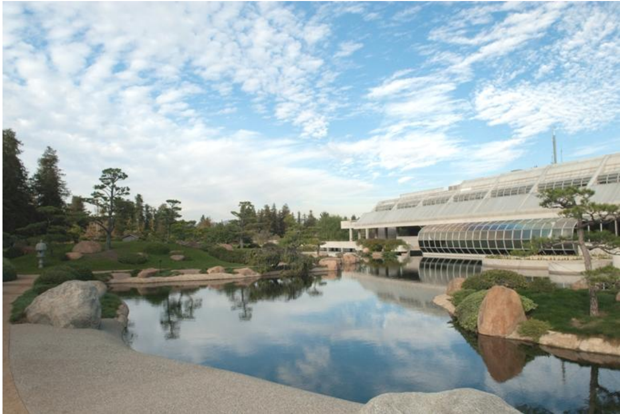
Donald C. Tillman Water Reclamation Plant
