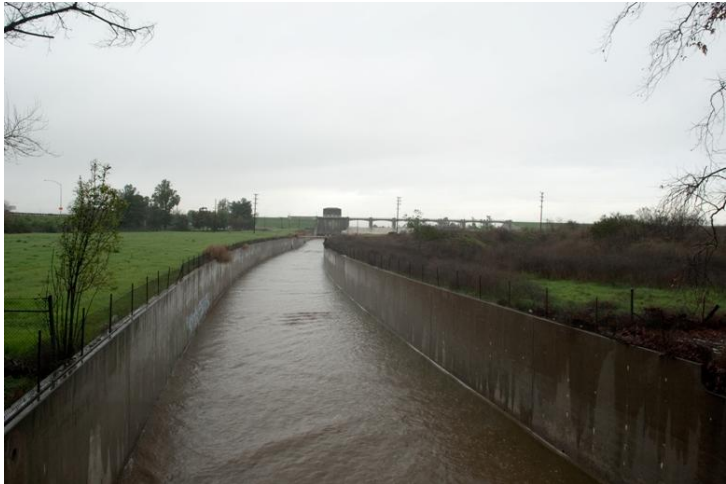
Sepulveda Dam and Channel
