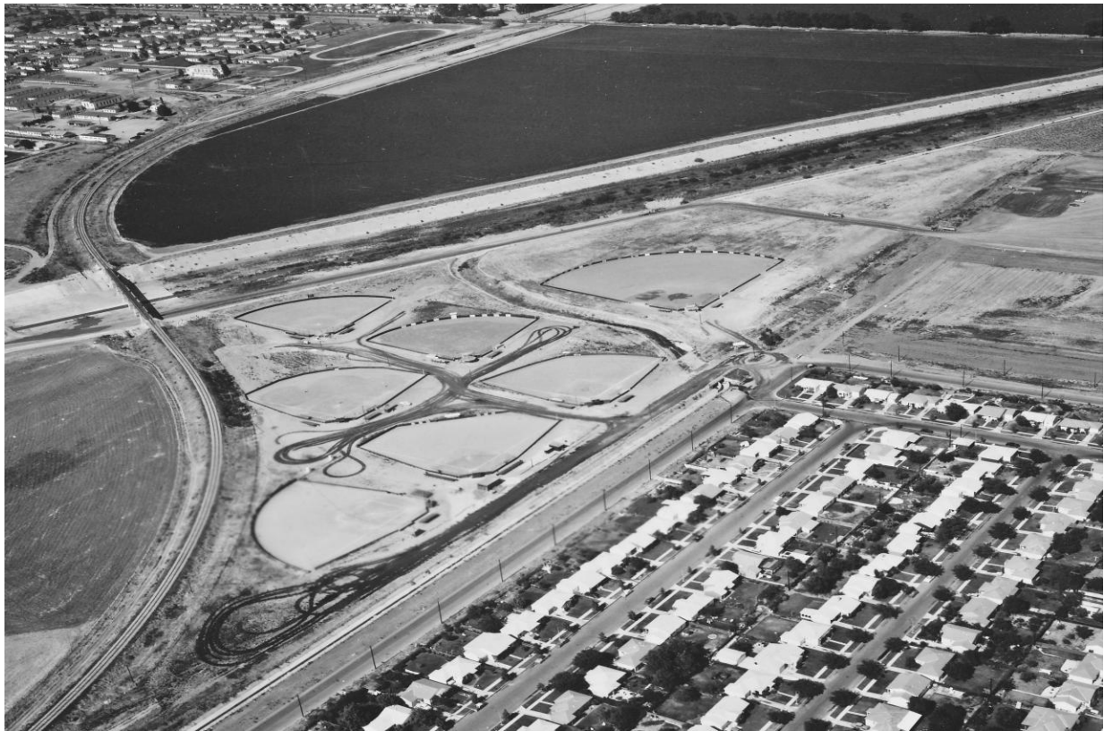
Sepulveda Ball Park Being Constructed, June 1955
