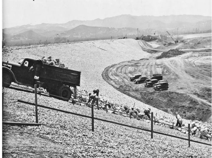
Sepulveda Dam Construction 1940
